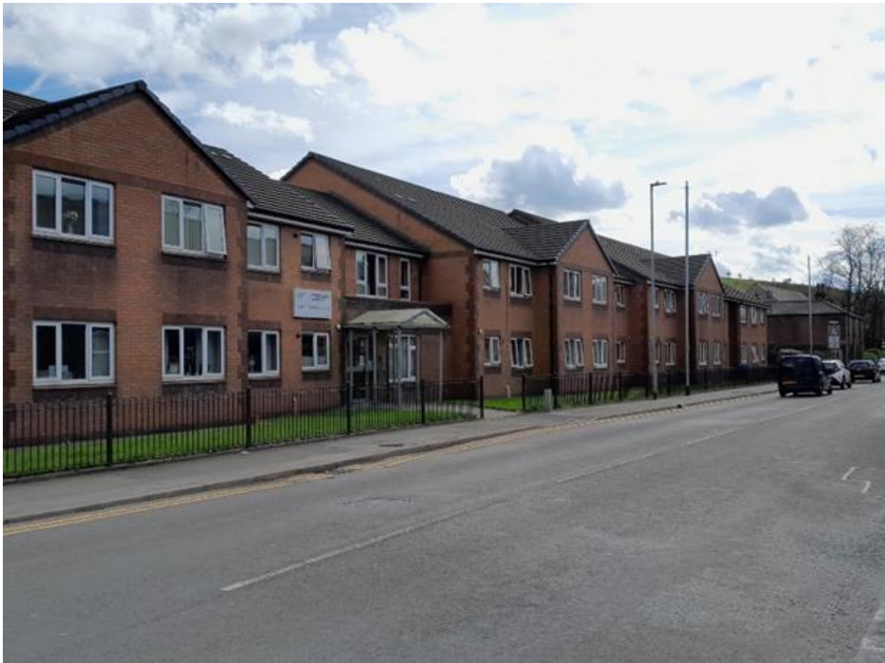
Figure 3.25 - Social housing in Rochdale
